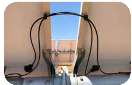
Routing around hazardous areas is one of the most important considerations. Module interface brackets are specific areas of danger, being areas of pinch points. HellermannTyton Solar Locking Clamp is installed in this photo. Part number 151-02501
